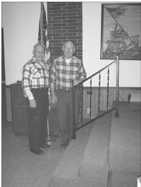
Bill Lyford and Charlie Mathey rebuilt the stage steps and added a hand rail for safety in response to the January 2006 VFW News article asking for volunteers to rebuild the steps. The original steps were set at different heights causing people to trip on them when ascending or descending the stage. Thanks guys! (Matt Klos photo).
