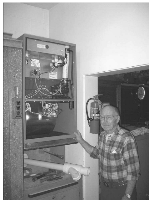
Charlie Mathey stands next to the upper hall furnace explaining how the venting would be tied into the meeting hall. This was the second high efficiency furnace installed to help heat the Post. (Matt Klos photo.)
