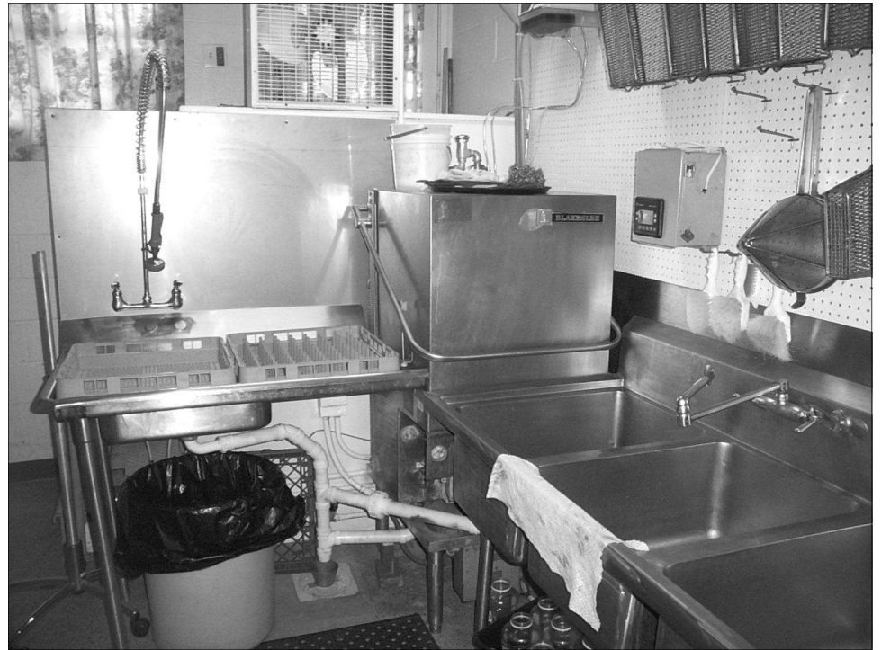
The automated dishwasher installed in the VFW kitchen, ready to tackle some dirty dishes. (Photo by Ralph Ritter).
