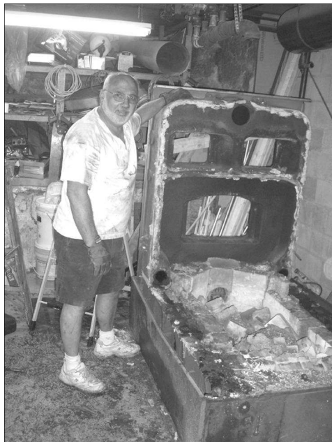
Ralph Ritter stands next to the boiler he, Charlie Mathey, and Bud Porter razed to make room for the energy efficient replacement boilers.
