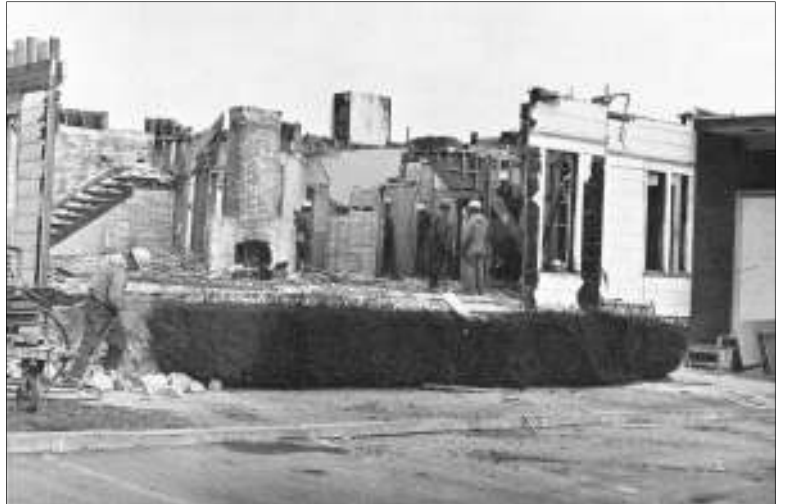
Demolition of the old Austin home, post headquarters in its early years. Work began on November 16. Workmen will take building to the first floor level, then erect siding, a roof and a new entrance at the corner of this area which will become one large room. 1972.
