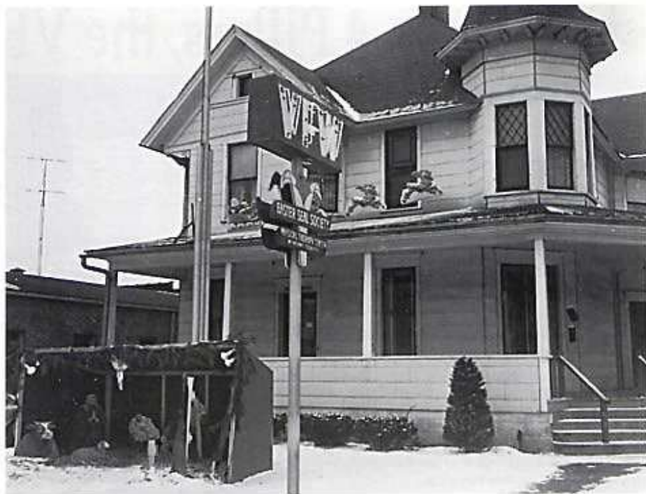
VFW MEMBERS PURCHASED this home from the Austin family, 240 Throop Street, for $12,000 and started building an addition in 1952. Joe Thiede was installed as Commander at the first major ceremony in our second floor meeting hall in 1954.
